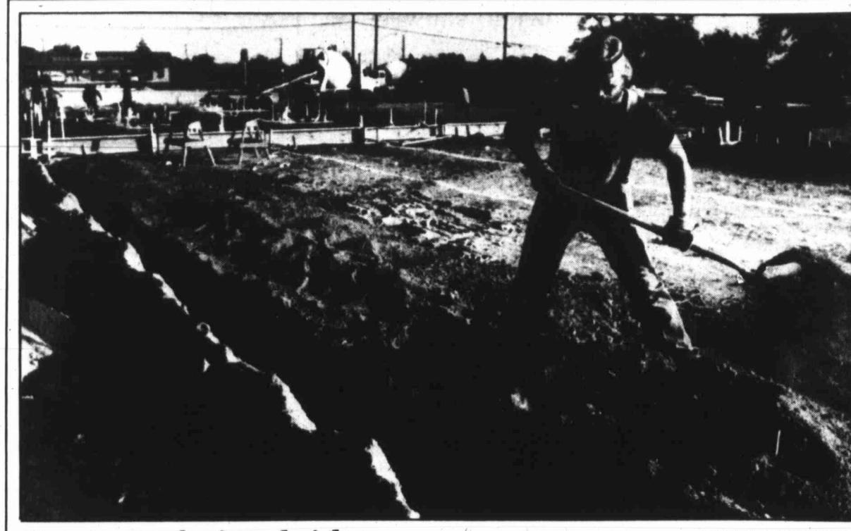
Concrete being laid Tom Smith of Ernest Herrera Construction shovels dirt away from the edge of a trench as concrete is being poured in the background as part of the new Comanche Trail Nursing Home located at the corner of Wasson and Parkway roads.
