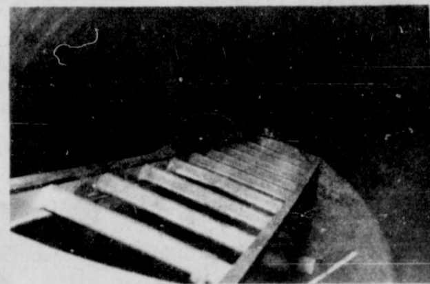
"The Hole" ...Two Trapped In Pit
