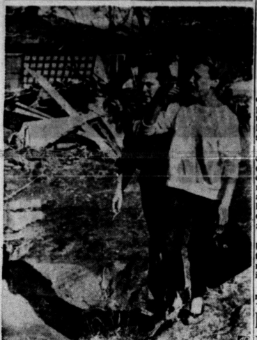
SEES WRECKED HOME THROUGH TEARS — Mrs. Leslie Behunin is in tears as she and her husband arrive back at the scene of Baldwin Hills Reservoir flood to find their home smashed by the rushing waters. "I have no home," she repeated. There was one of hundreds destroyed or damaged by the waters. (AP Wirephoto)
