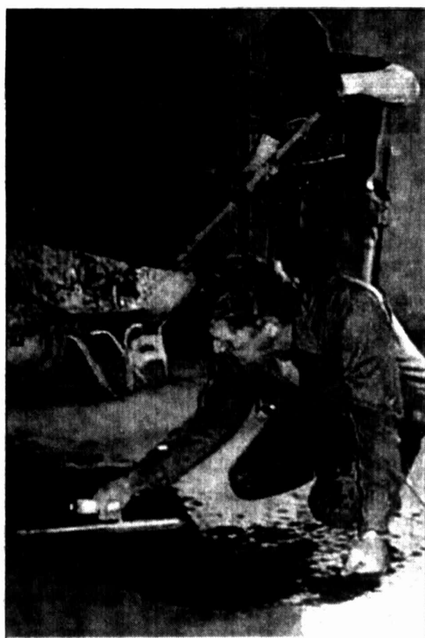
HERALD photos/Marsha Sturdivant Projected completion for Big Spring Junior High School is April. Above, Luther Chavez, left, along with Daniel Byars and Michael Perkins of Stallford Flooring, install maple flooring in the east gymnasium. At right, Doug Tatum smooths wet cement onto the stage area floor with the assistance of David Villareal of Monterey Construction. And below, Stephen Burton, of Stover Electric, checks the installation of a two-and-a-half-gallon water heater under a sink in the work area off the library.
