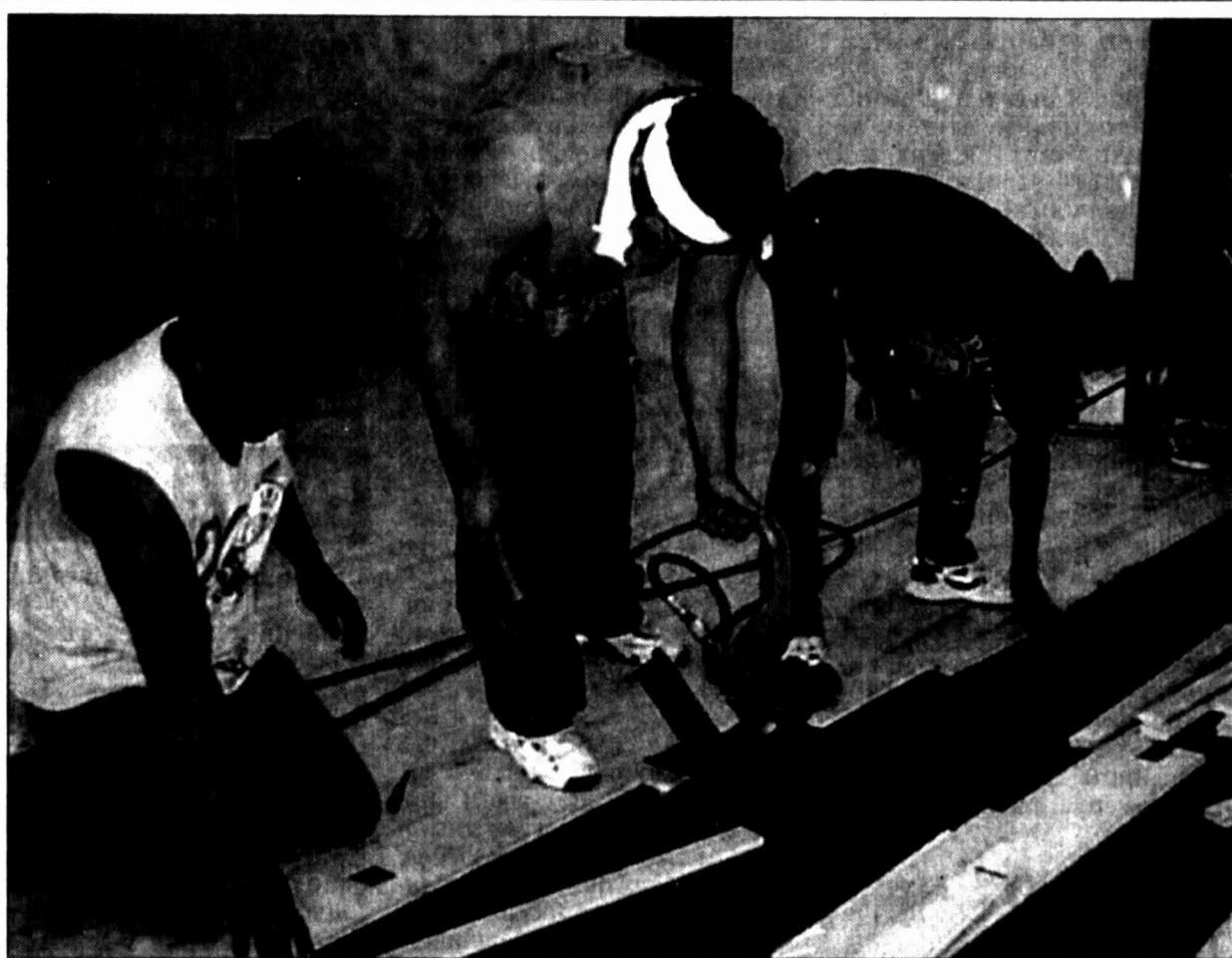
HERALD photos/Marsha Sturdivant Projected completion for Big Spring Junior High School is April. Above, Luther Chavez, left, along with Daniel Byars and Michael Perkins of Stallford Flooring, install maple flooring in the east gymnasium. At right, Doug Tatum smooths wet cement onto the stage area floor with the assistance of David Villareal of Monterey Construction. And below, Stephen Burton, of Stover Electric, checks the installation of a two-and-a-half-gallon water heater under a sink in the work area off the library.
