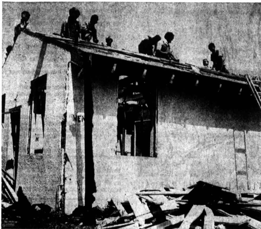
STUDENTS AT WORK — Students in the Big Spring High School vocational building trades class are busy rebuilding storage and restroom facilities at the baseball park as part of a class project. The boys are learning the fundamentals of the carpentry trade and can be rated as second- or third-year apprentices on graduation from high school.
