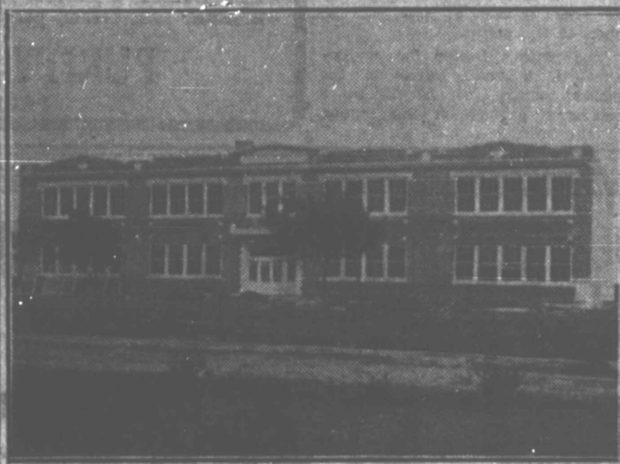
The Portales Junior High school was erected in 1929 at a cost of $25,000. Two units have been added to take care of demands since that date. They cost $14,000. Enrollment in Junior high is astoundingly high. (Picture from News Magazine).
