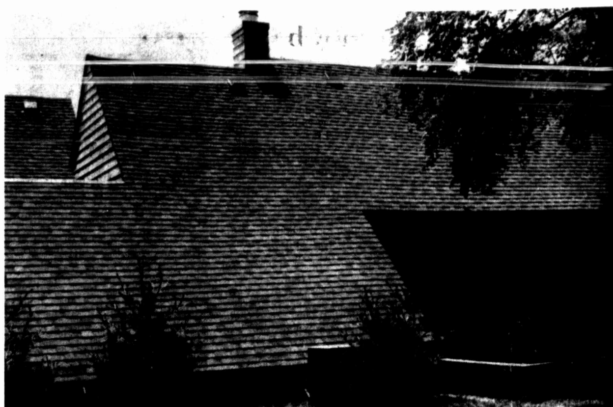
Though this is a new home, it emphasizes the role that the roof plays in both protection and exterior design. The roof of attractive asphalt shingles serves to enhance the design of this contemporary home.
