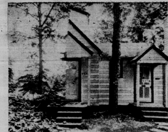
NOW JOE'S GOT HALF A HOUSE—This is what is left of Joe Conrad's house in Charlotte, N. C., after a wrecking crew split it down the middle to make way for a new street. Conrad had objected to condemnation of his property. He lost that battle, but insisted the city could take only half his house. So workmen sawed it in two. Conrad says he'll remodel what's left and rent it for offices. (AP Wirephoto)
