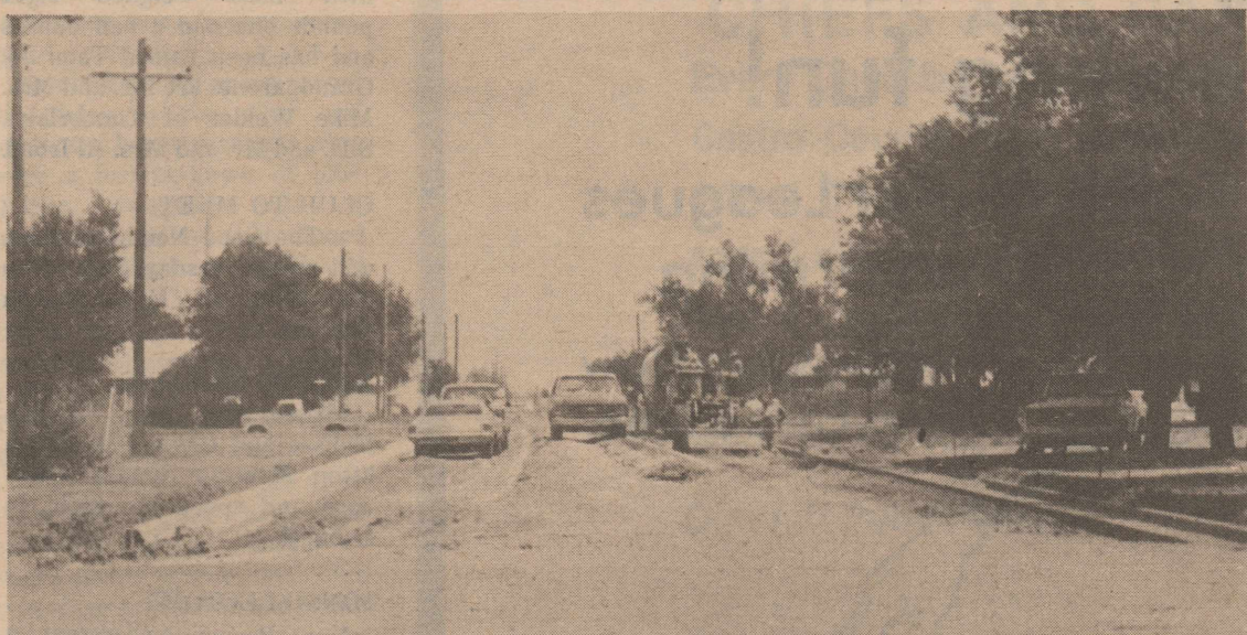
PAVING WORK CONTINUES - Streets in the city are the focal points of activity as the paving project progresses. This photo, made at the intersection of Hart schools recently, shows one of the busiest streets in the city is not ready for the beginning of school. (Staff photo)
