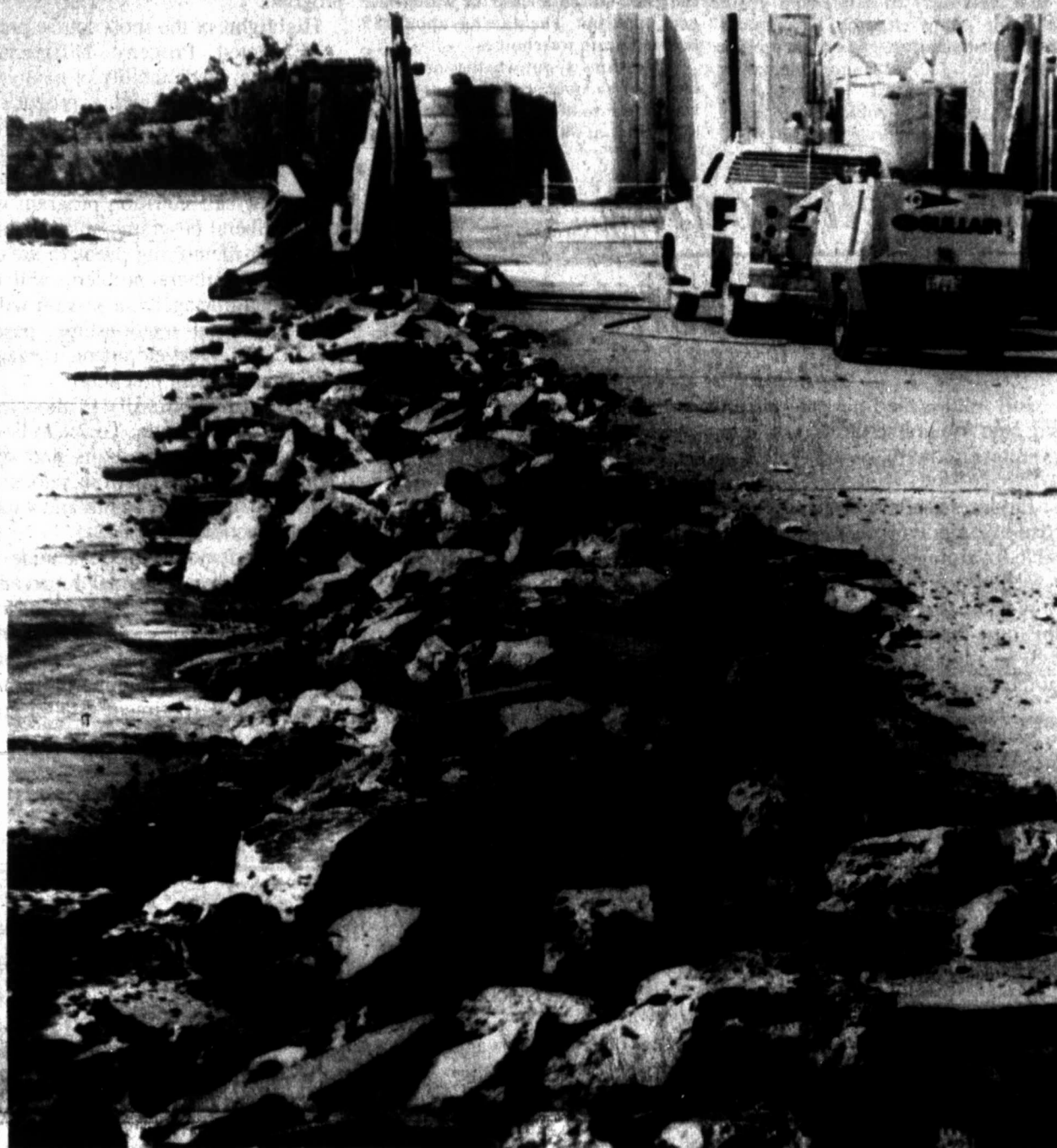
BUSTIN' PAVEMENT - Oak Street in the downtown area is taking on a new look as the city prepares to install a new eight-inch water line to provide better water service for the area. City crews have been breaking through the pavement as the project gets underway.
