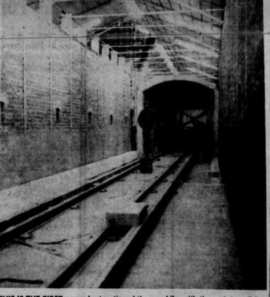
THIS IS THE FIRST, or pre-heat section of the new kiln, with the roofed, or firing section seen in the background. A third section, the cooling section is on beyond. Capacity of each section is 30,000 bricks for an overall capacity of 90,000 bricks. 30,000 per day can be produced when the kiln is finished. Southwestern Brick and Tile has applied for a patent on this kiln which has the advantages of a tunnel kiln without the disadvantages of the old-style tunnel which had to be a continuous operation. The firm's products of standard bricks, Romans, Normans, tile and patio pavers can be produced in this kiln.
