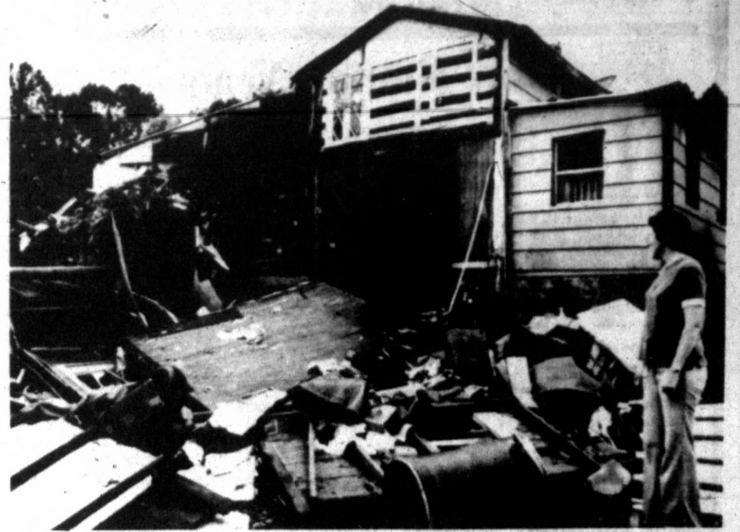
A 63-YEAR-OLD MAN died in the collapse of this home Wednesday in Great Falls, Va. The house collapsed during a tornado spawned by the remnants of Hurricane David.
