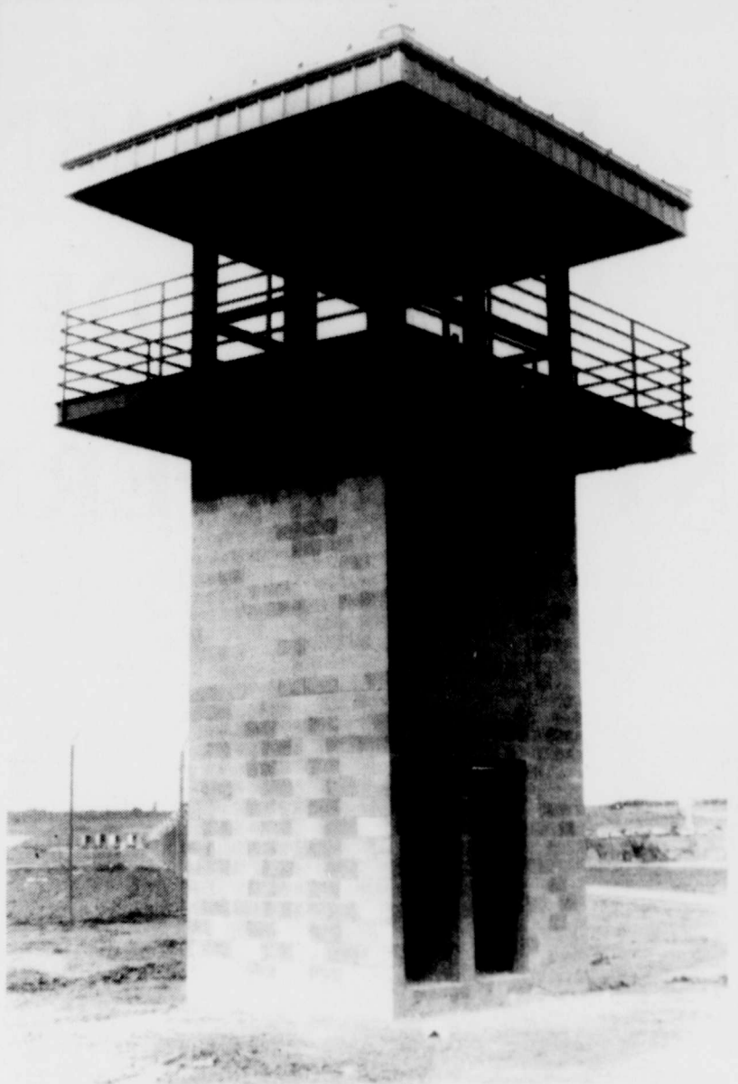
PICKET IS TOPPED: Workers put the top on the picket located just outside the fence at the 80-John Wallace Unit this week. Work is on schedule for a mid-May completion date said Texas Department of Corrections officials.
