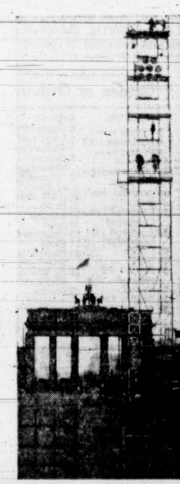
WATCH TOWER —New watch tower is built of steel piping and supports a camera and sparse crew. It is keeping a watchful eye on doings in East Berlin.
