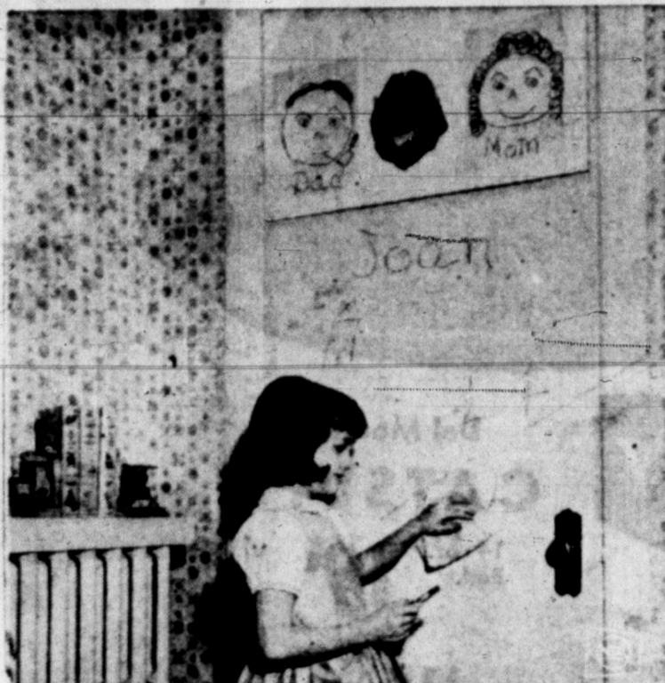
King-size scribbling space is offered by a door sheathed in plastic-finished hardboard. Composition board, top, takes thumbtacked pictures and messages.
