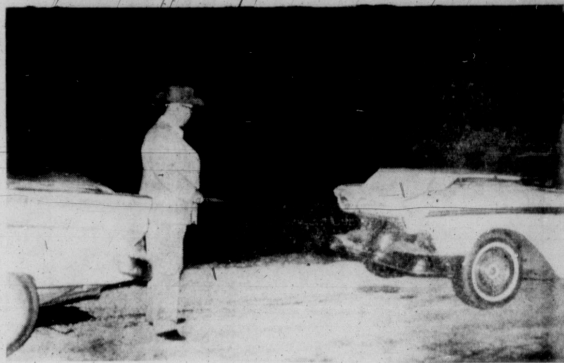
Interstate 20 Bridge Wreck
