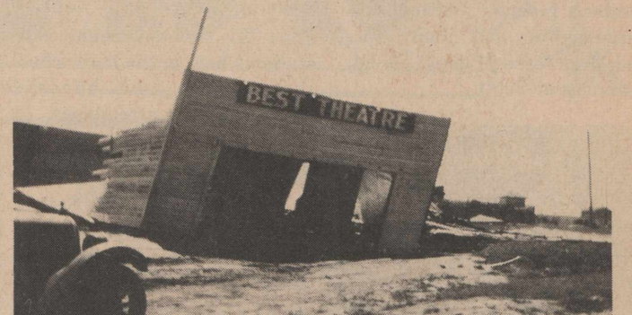
OLTON'S FIRST THEATER, destroyed in 1929 when a tornado slashed through town, is pictured here following the storm. (Personal photo of Mrs. Paul Burrus)
