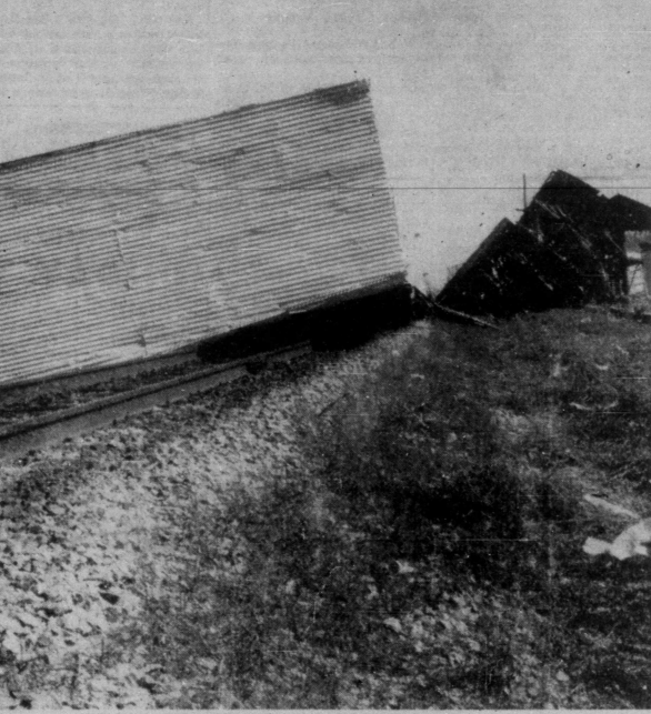
RAILROAD BLOCKED —This is another view of the wind-wrecked building which came to rest across the main line track of the Santa Fe Railway.
