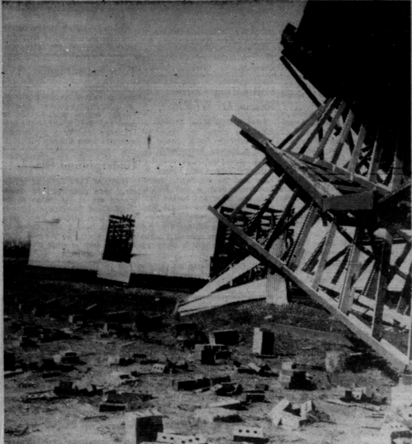
BUILDING UPROOTED —Strong wind gusts left this debris as they uprooted this structure formerly used by Walter Hales Lumber Co. on the East Highway. Gusts were hitting as high as 50 miles per hour when the building toppled.
