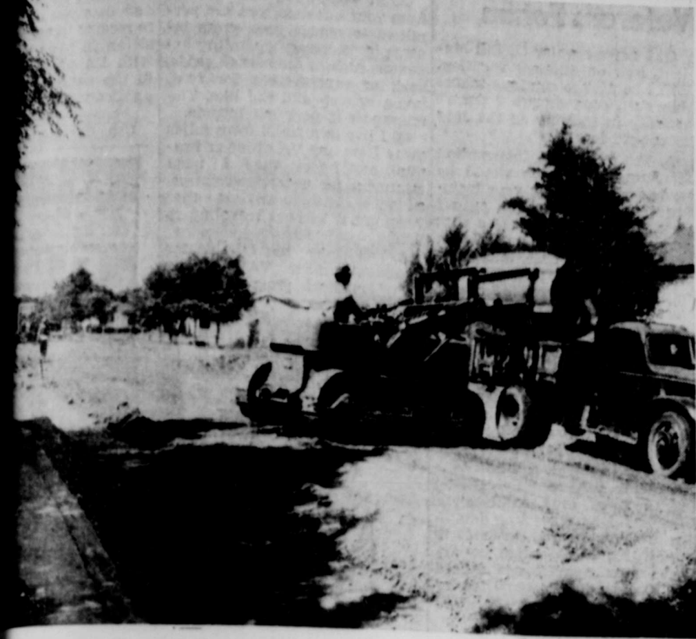
ON DRAKE—The 1000 block on South Drake is being paved this week, with some curb being poured. The city has contracted the construction to the O. C. Watson Construction Co. The picture above shows some of the excavation work being done Tuesday.
