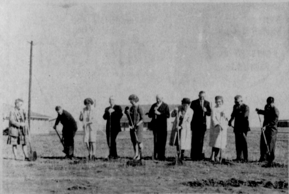
GROUND BREAKING---Officials and representatives of the local Methodist Church broke ground Sunday for the new church parsonage at 11th and Linn streets. Breaking ground were the Rev. and Mrs. Wesley Daniel, David McClellan, Mrs. Garland Head, George Buzzard, Mrs. Jack McWhirter, H.H. Crooks, Mrs. T.D. Sansing, Garland Head, Mrs. Bruce Sheets, Jack McWhirter and Frank Buzzard.
