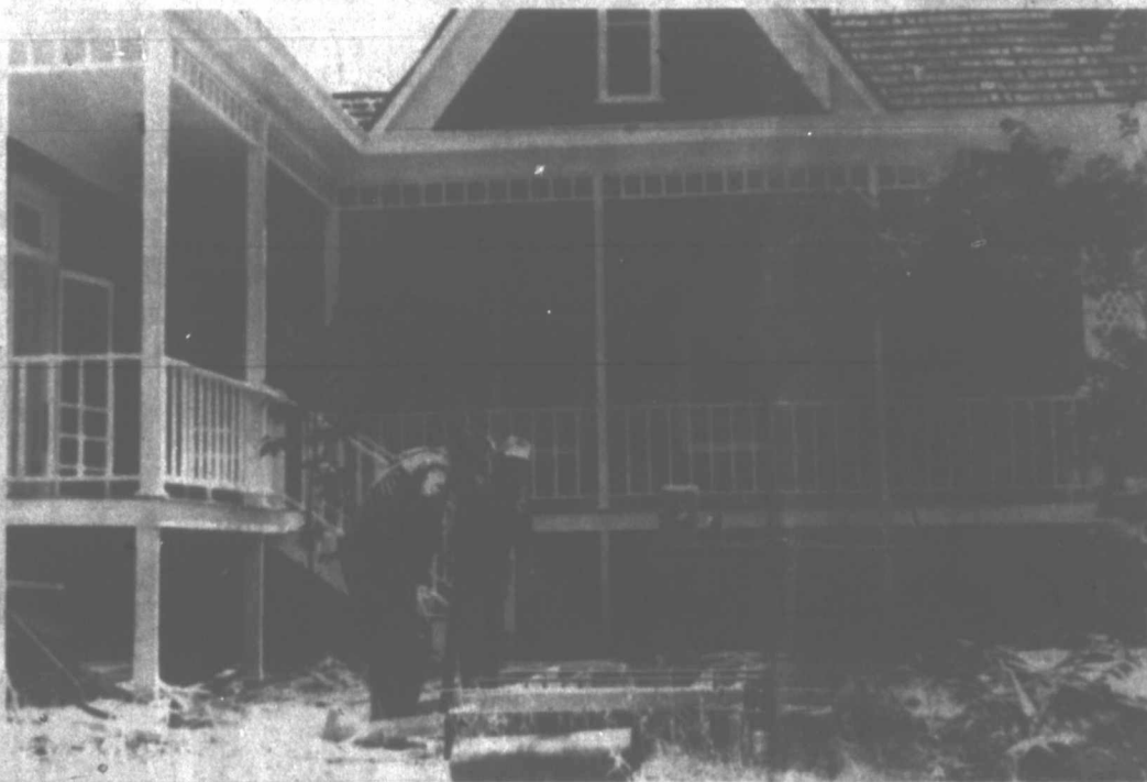
THE HERITAGE HOUSE on Chestnut Street in Colorado City is nearing completion for the Open House scheduled for the last Sunday of August. Gerald Frizzell and Tony Espinoza are shown here repairing the cellar in the back yard.
