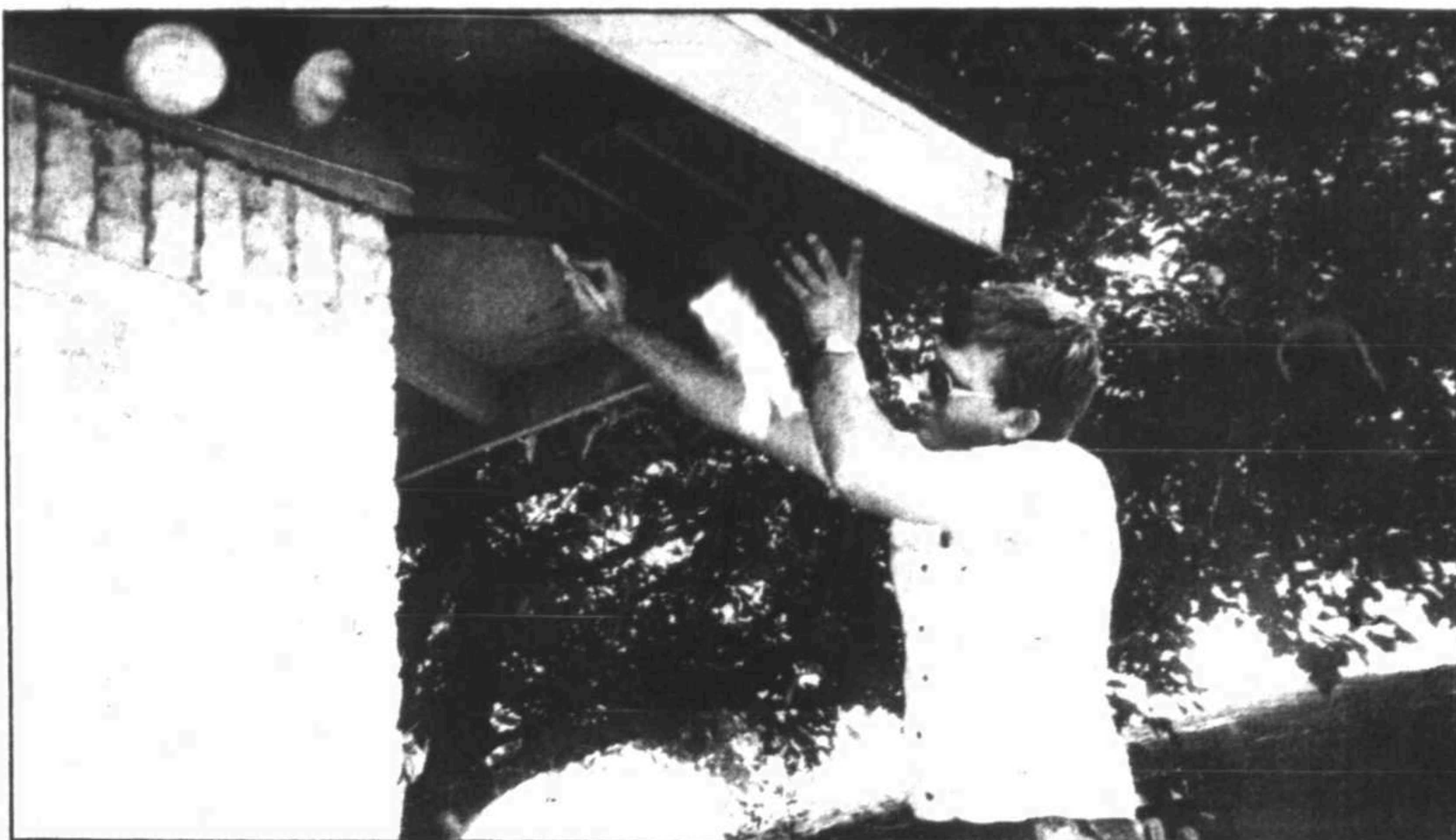
An expert installer from Mid West Door and Window fits new steel siding on to this
