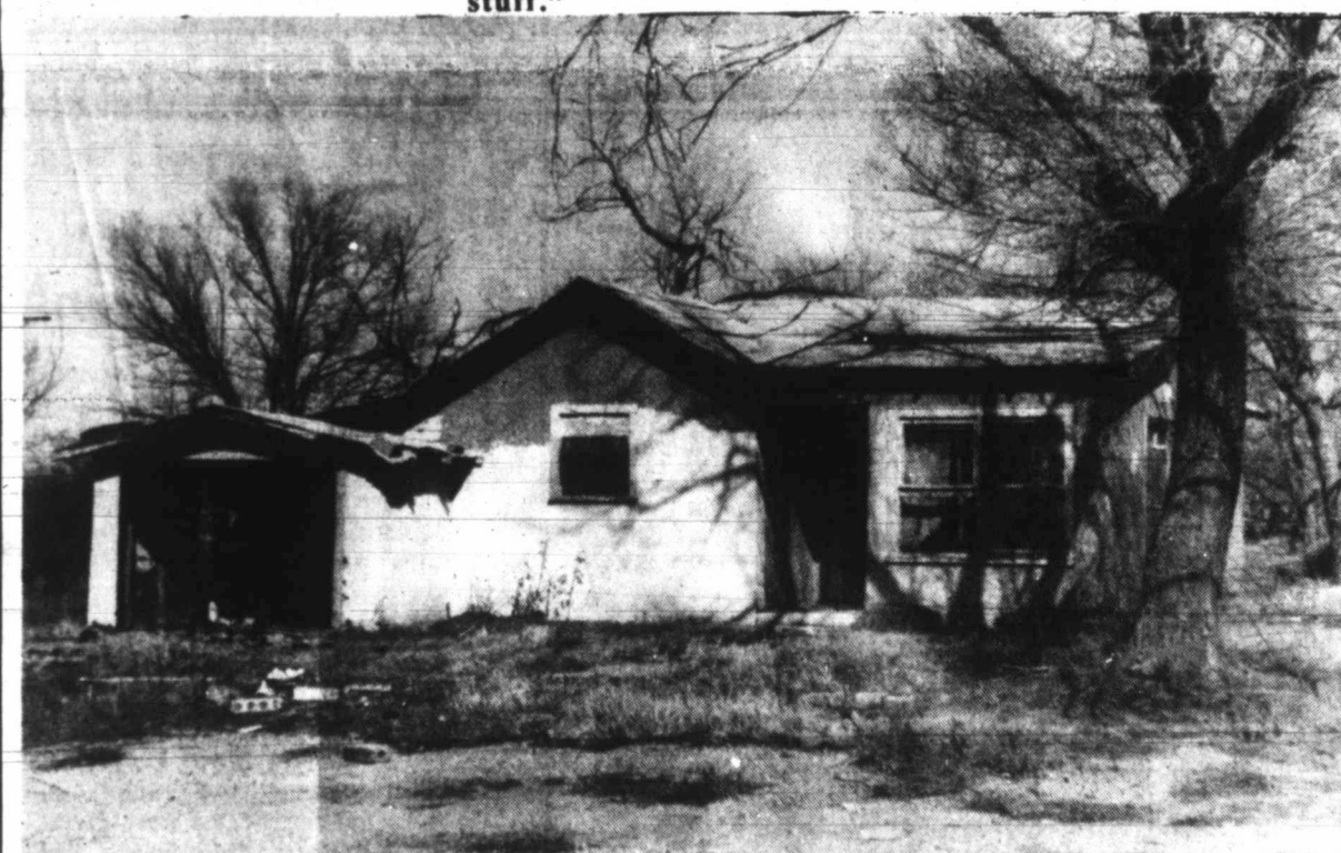
SLATED FOR DEMOLITION....This house, located at the corners of 4th and Cherry Streets is scheduled to be torn down early this week.
