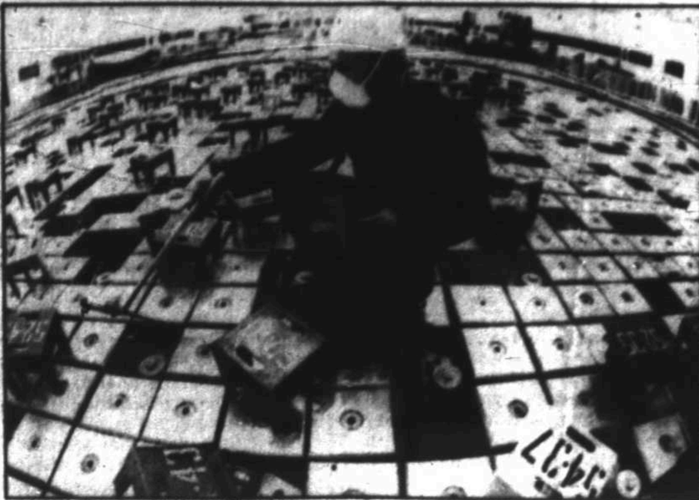
Soviet worker V. Gladenko, wearing a surgical cap and mask, measures the radiation level in what Soviet officials identify as the upper part of reactor No. 1 at the Chernobyl nuclear power plant.
