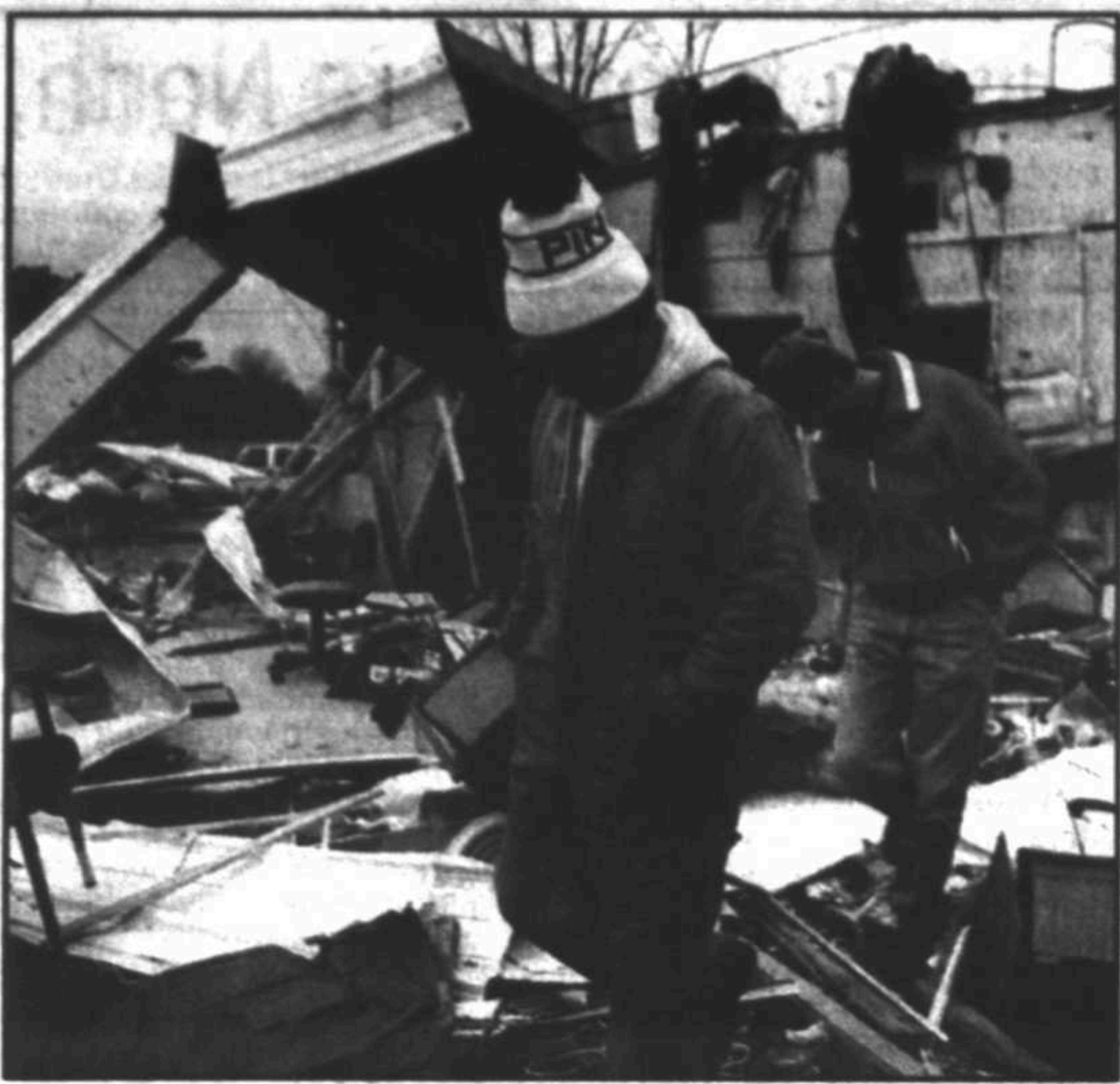
Employees waded through debris that once made up the car dealership in Sylamore, Arkansas, Monday. The tornado tore up this small Ozark town and left seven dead in its wake.
