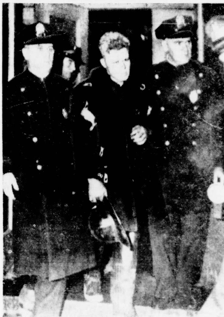
An unidentified fireman is helped from a Brockton, Mass., theater after a balcony fell killing 10 of the 20 men who were fighting an early morning blaze. The roof of the theater had been weakened by ice, snow and fire. (NEA Telephoto.)
