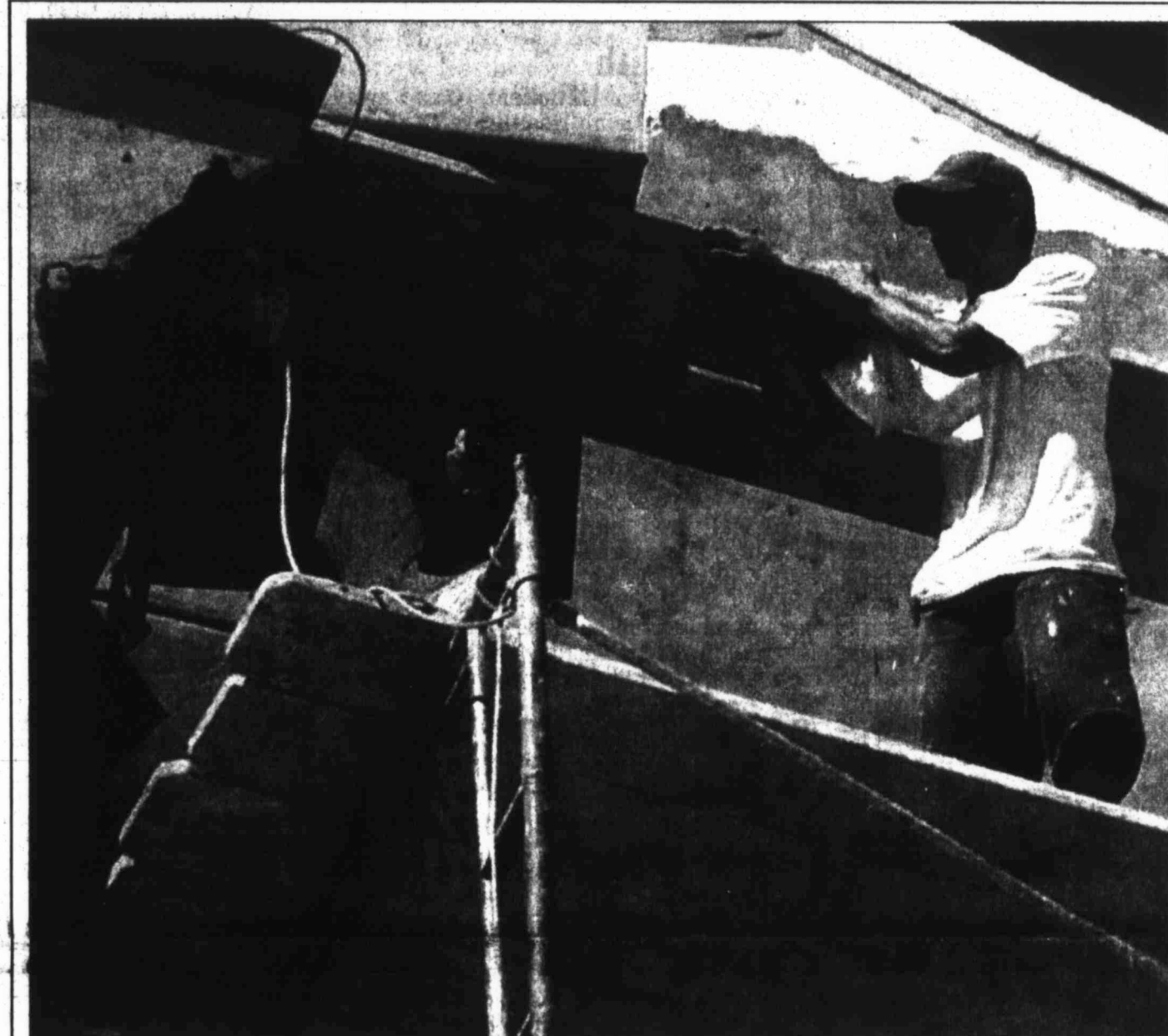
Construction workers were busy Saturday doing stucco work on the new Holiday Inn Express being built at the intersection of Interstate Highway 20 and U.S. 87. Barring any weather problems, the hotel is expected to be completed by the end of next month.
