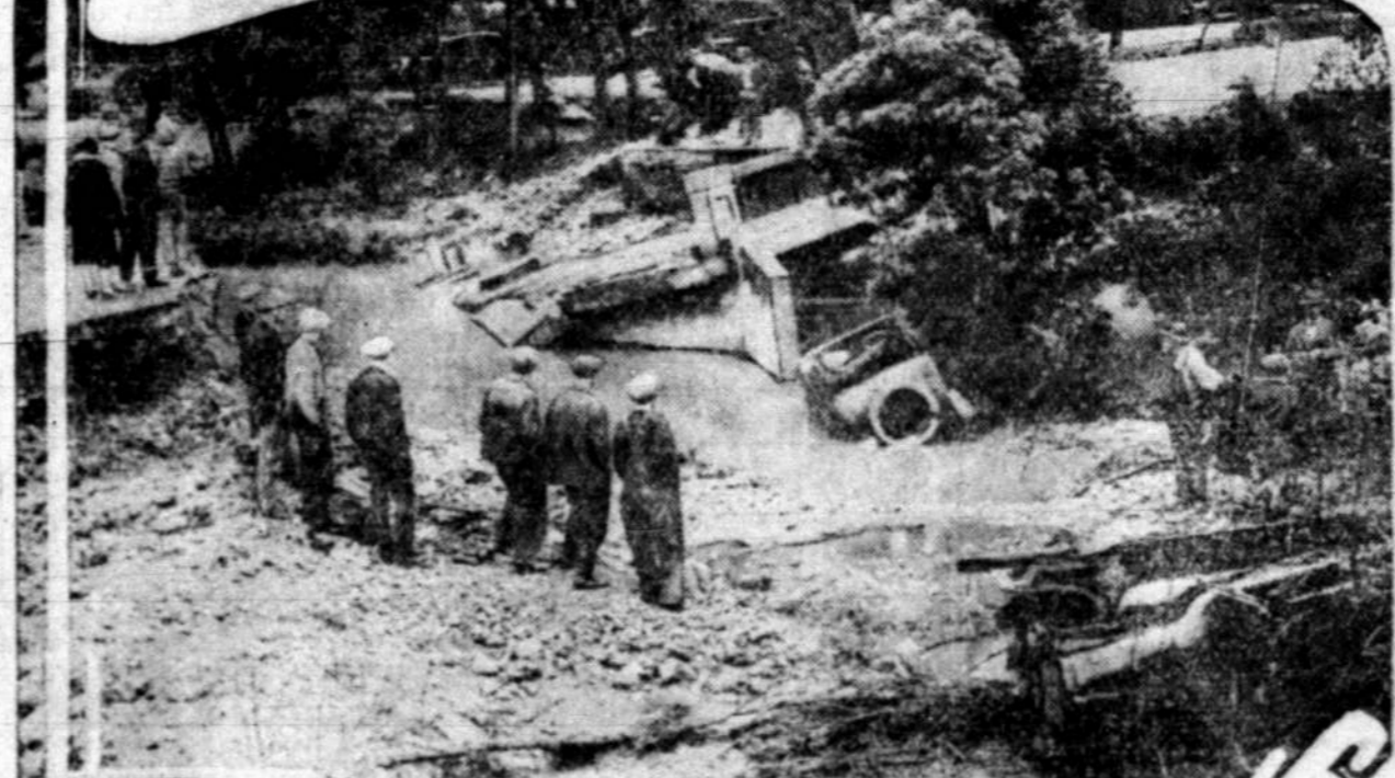
Northern Illinois, especially in Rockford and vicinity, was hard hit by a cloudburst which rapidly swelled the streams and caused floods that did a lot of damage. The illustration shows a scene on the state highway between Rockford and Detroit, Wis.
