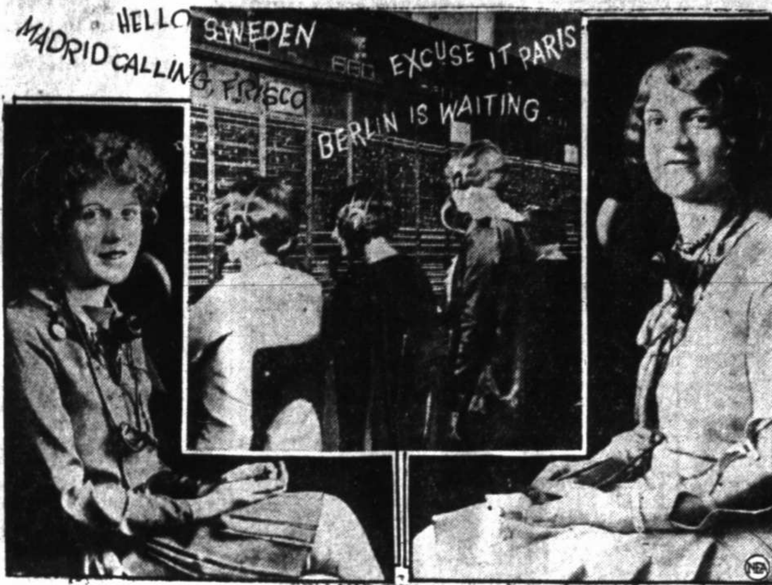
How awfully thrilling, these trans-Atlantic telephone operators will tell you, to chatter with friends in London. Pretty Alice Frazer, left, and Margaret Lang, right, have talked with many world celebrities, too. Center is a view of the switchboard in New York, through which all calls are routed.
