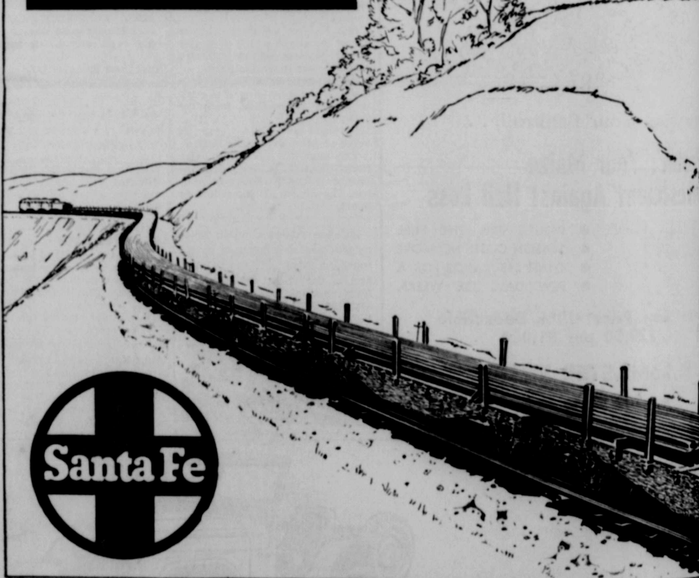
Quarter-mile lengths of welded steel rail curve around a foothill like wire cable.
