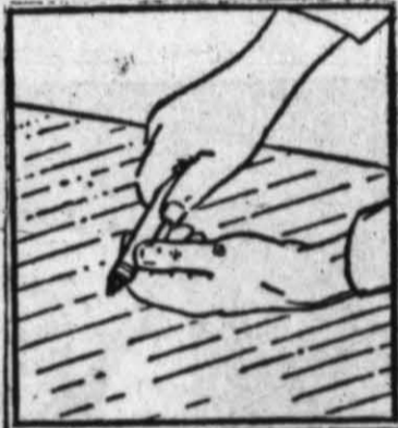
TALCUM POWDER or powdered graphite puffed into cracks sometimes silences milk squeaks in a floor.
