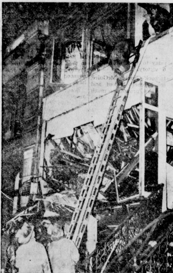
TWO DIED HERE—When fire-weakened upper floors of this New York building collapsed while the flames were being brought under control, two fire insurance company patrolmen were trapped and died where they fell. Here firemen probe the remains of the building for possible unknown victims.
