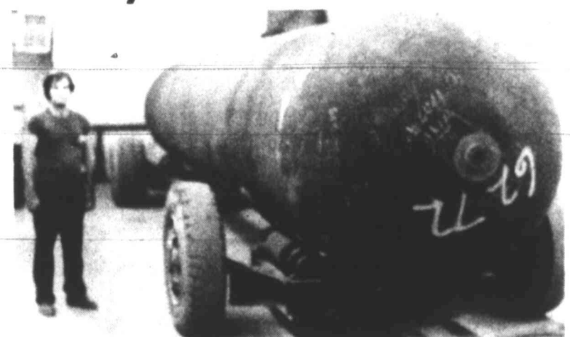
TAKING PICTURES — The tank are X-rayed again and again until every flaw is removed. Then they are baked at temperatures above 1,000 degrees to remove stress.
