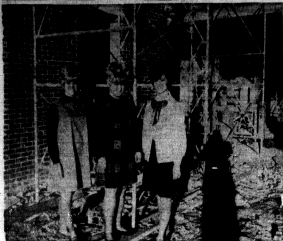
LOOKING AT a new girls' dorm under construction at Panhandle State College are, left to right, Georgiann Grayson, Pampa; Jan Lee, Perryton; and Sherry Mahaney, Dalhart. The new girls' dorm is scheduled to open in September, 1969. The college is located in Goodwell, Okla.
