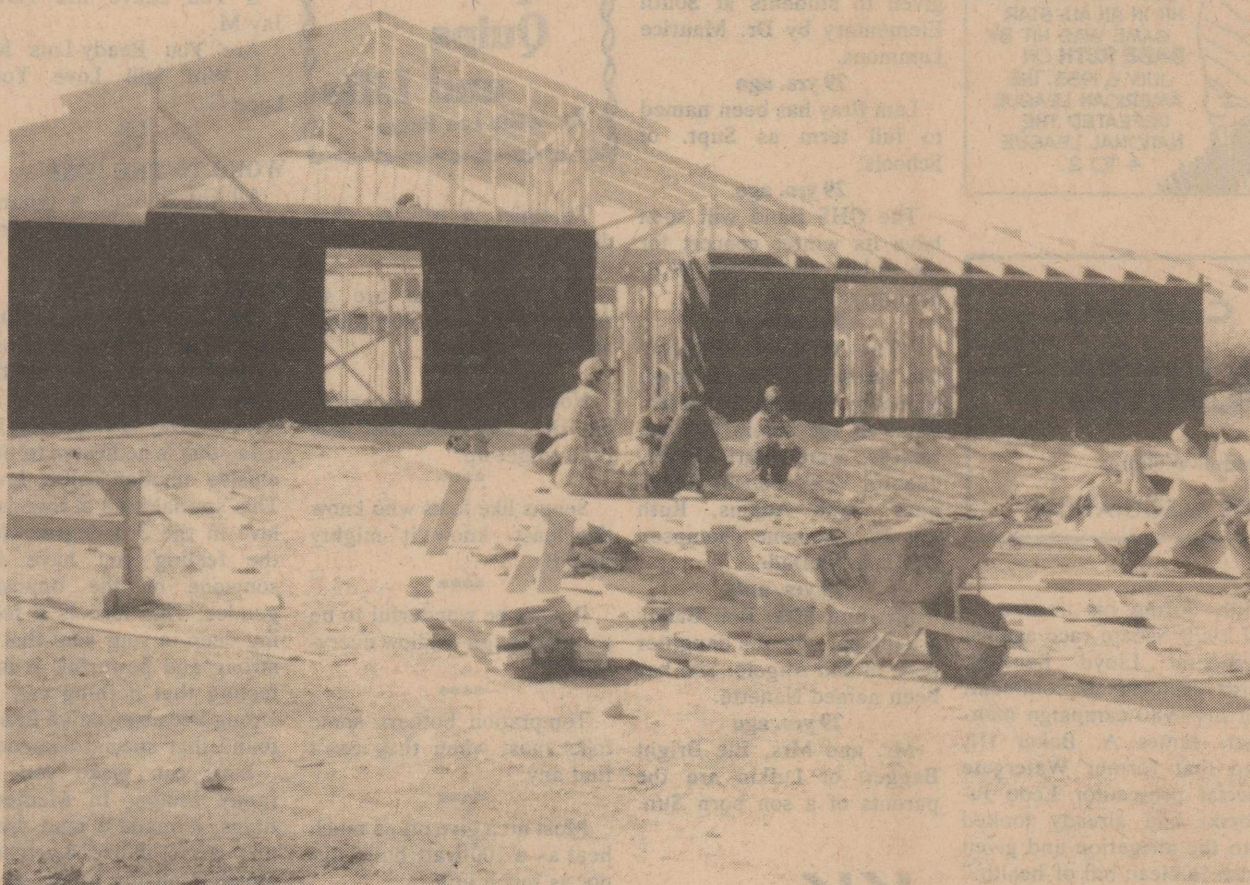
HOME CONSTRUCTION BOOMS in Ozona. Mr. and Mrs. Johnny Jones will make this house their home when it is finished on the west hill. Also nearing completion on Mitchell Hill is the new home of Mr. and Mrs. Bill Mason. Mr. and Mrs. Tom Cameron's new home in Country Estates
