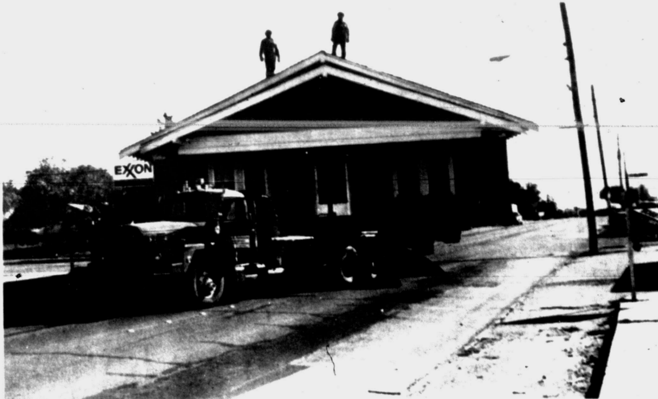
HOUSE MOVING — This house was being moved Tuesday morning from 2312 Ave. M to the Bullard Ranch, located west of town. The house was built by Jean Bullard's grandparents, Joda and Vashti Monroe, in the early 1900s. (SDN Staff Photo)
