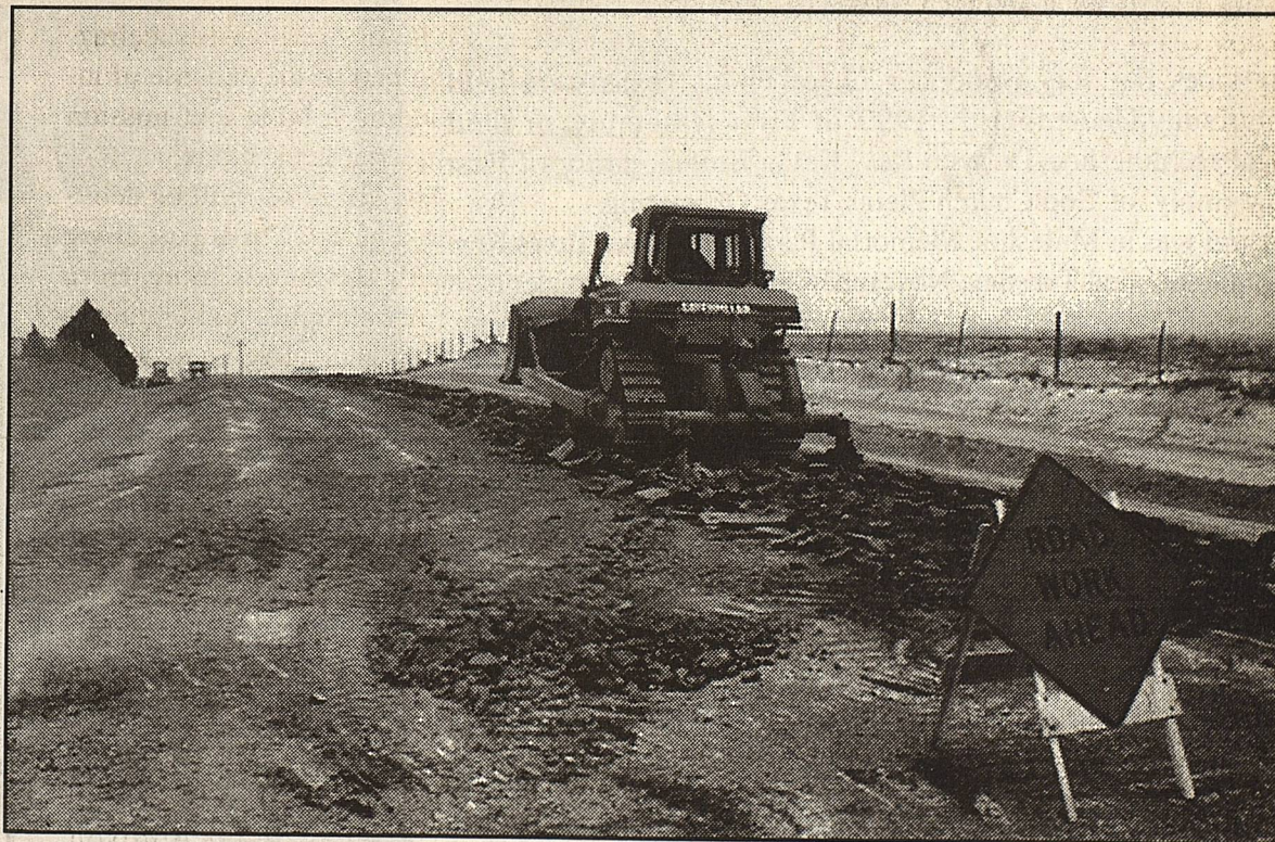
Pct. 3 employee Hershell Smith operating a dozer ripping up asphalt on road
