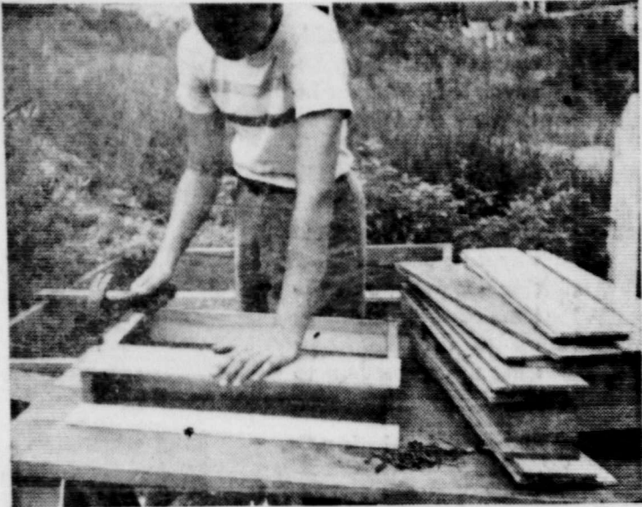
Flats come "knock-down" and are put together with a few nails.
