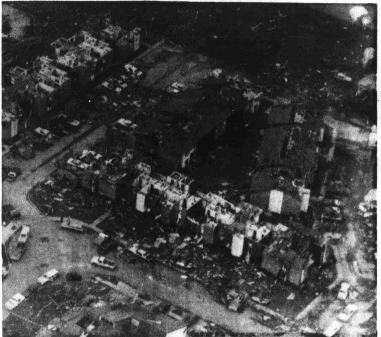
TORNADO DAMAGE — This airview shows extensive damage in Wichita Falls, Texas caused by a tornado that ripped through the city late Tuesday.
