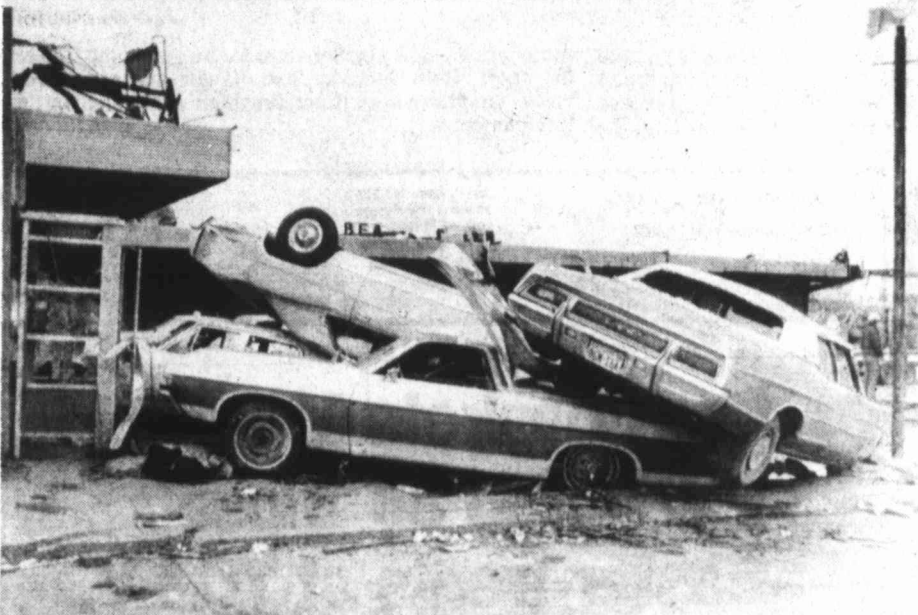
STACKED LIKE TOYS — Automobiles in a shopping center in Wichita Falls, Texas were stacked like toys after a tornado ripped through the city Tuesday.
