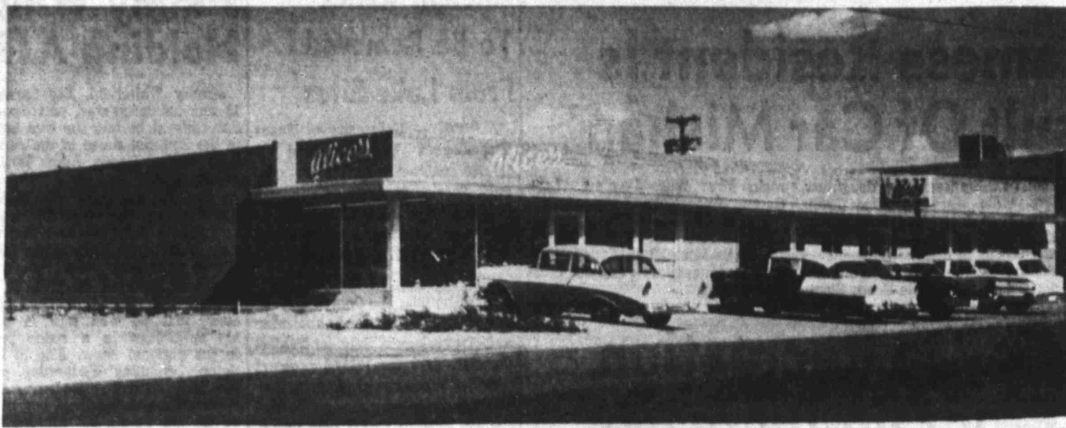
NEW SHOPPING CENTER ... Elliott Building Near Completion
