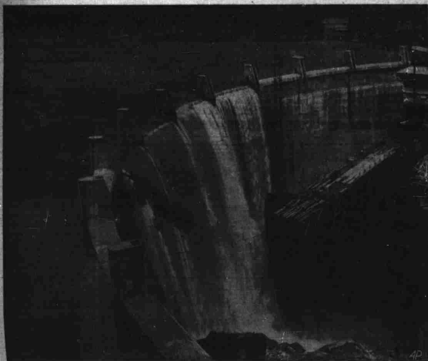
DAWN OF NEW DAY FOR HYDRAULIC MINING may bring a gold boom to land around Auburn, Cal., where this concrete barrier 125 feet high crosses the American river, as the first of a series of debris dams being built under the direction of army engineers. Before hydraulic mining was legislated out of existence in 1893 after years of strife between miners and farmers, it produced the bulk of the gold mined in California. The lake is intended as a settling basin for sludges unworked for years.
