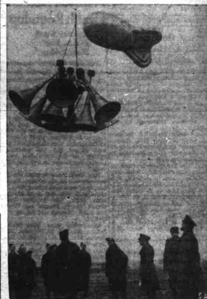
OUT OF THE CLOUDS a warning voice will come to tell Britons of air raid dangers. That's the theory which led to above demonstration of England's much-discussed balloon barrage near London. The speakers have a range of five miles.
