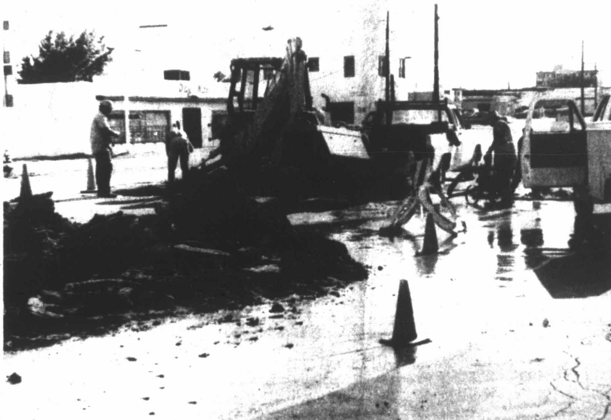
WATER LINE BREAK —The City's new backhoe/loader got a good workout last Tuesday when the water department crew had to dig through six inches of asphalt and eight inches of concrete to repair a split in an eight inch main water line at the busy intersection of Hickory and Second streets.
