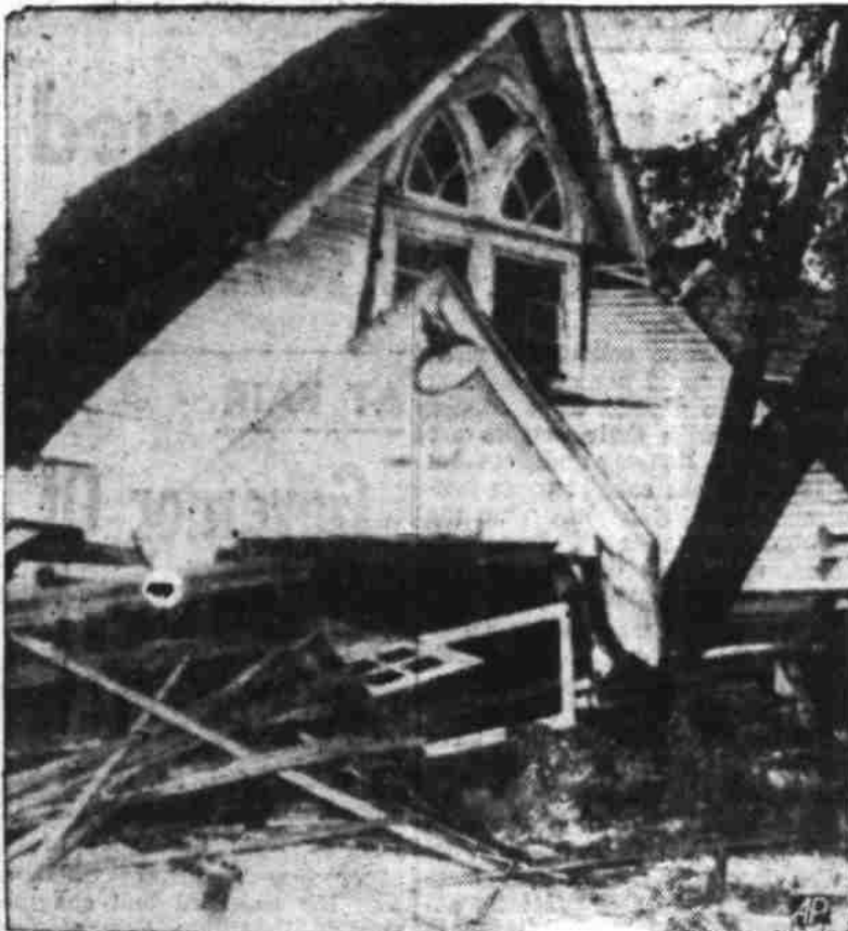
DAMAGED BY HURRICANE — A hurricane which swept in from the Atlantic Ocean flattened the Trinity Church on Tybee Island (Savannah beach) near Savannah, Ga. No one was in the church at the time and most of the island's 1,500 residents had been evacuated. (AP Wirephoto).
