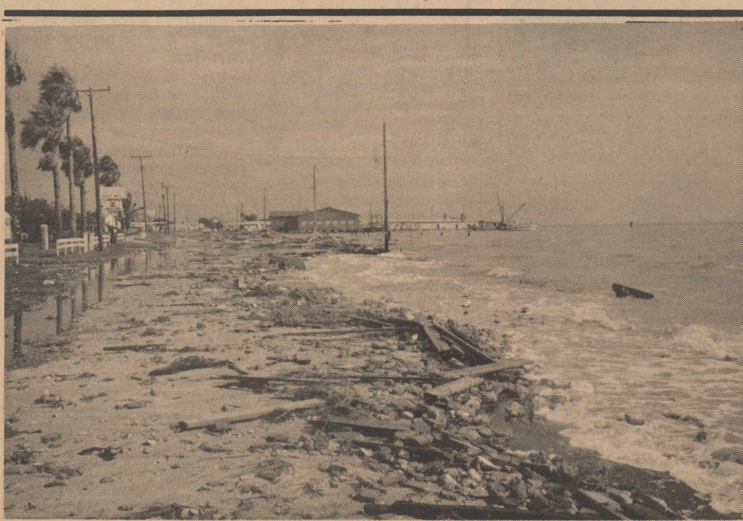
FERN DEVASTATION — Looking north along Fulton Beach Road toward the Paws and Taws Building, this photo illustrates typical damage caused in some local areas by the high tides, strong wind and lashing waves. Pilot Staff Photo.
