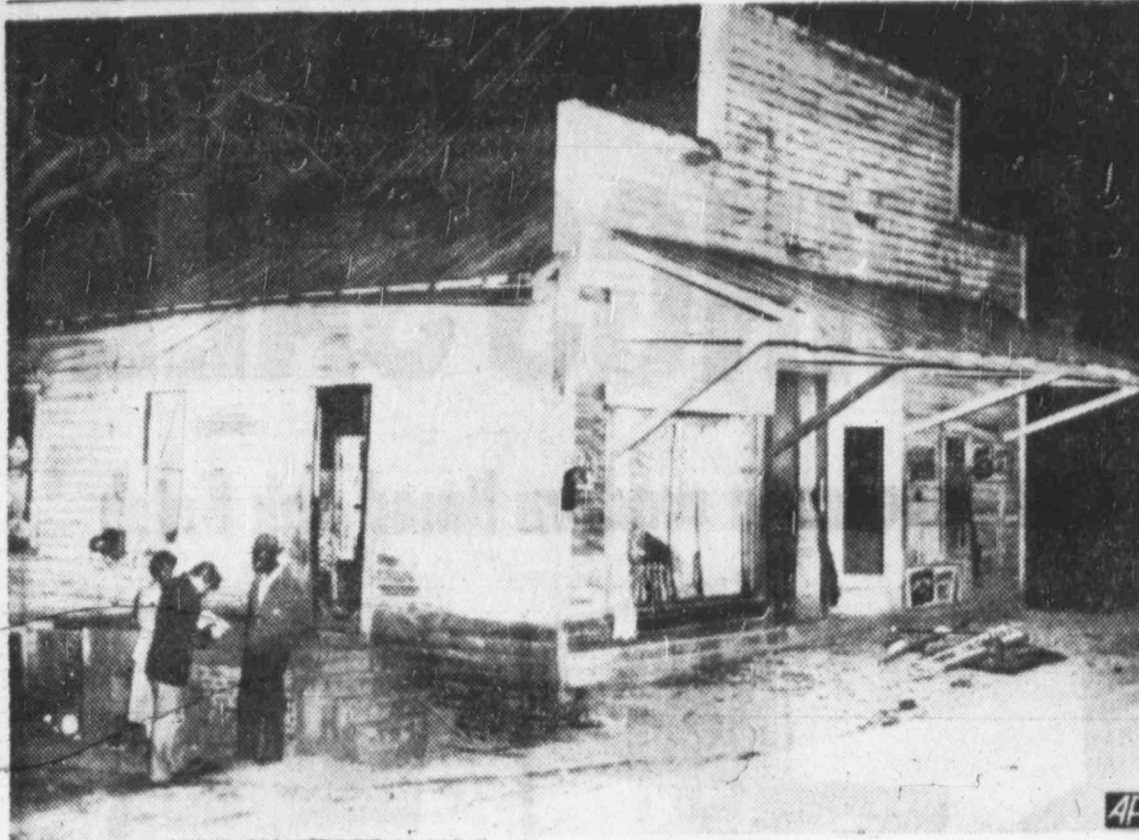
Blast Wrecks Building
