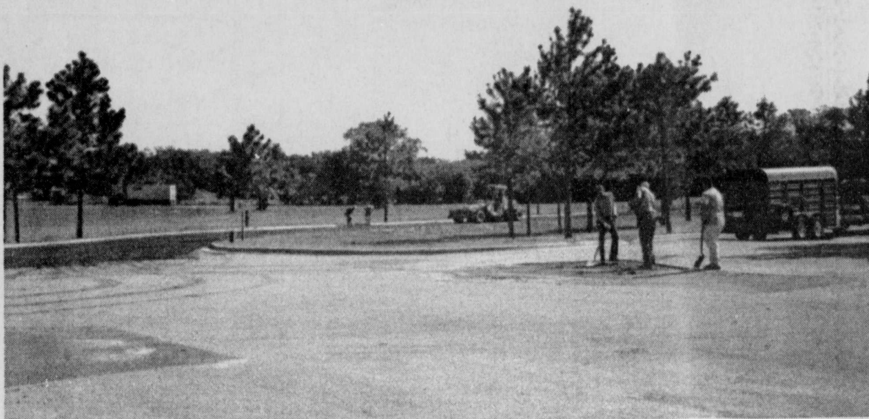
PRAIRILAND ENTRANCE GETS A FACELIFT as contractors prepare asphalt and new curbs down the driveway. They are patching the potholes and resurfacing the area. (Staff Phot by Liz Irwin)
