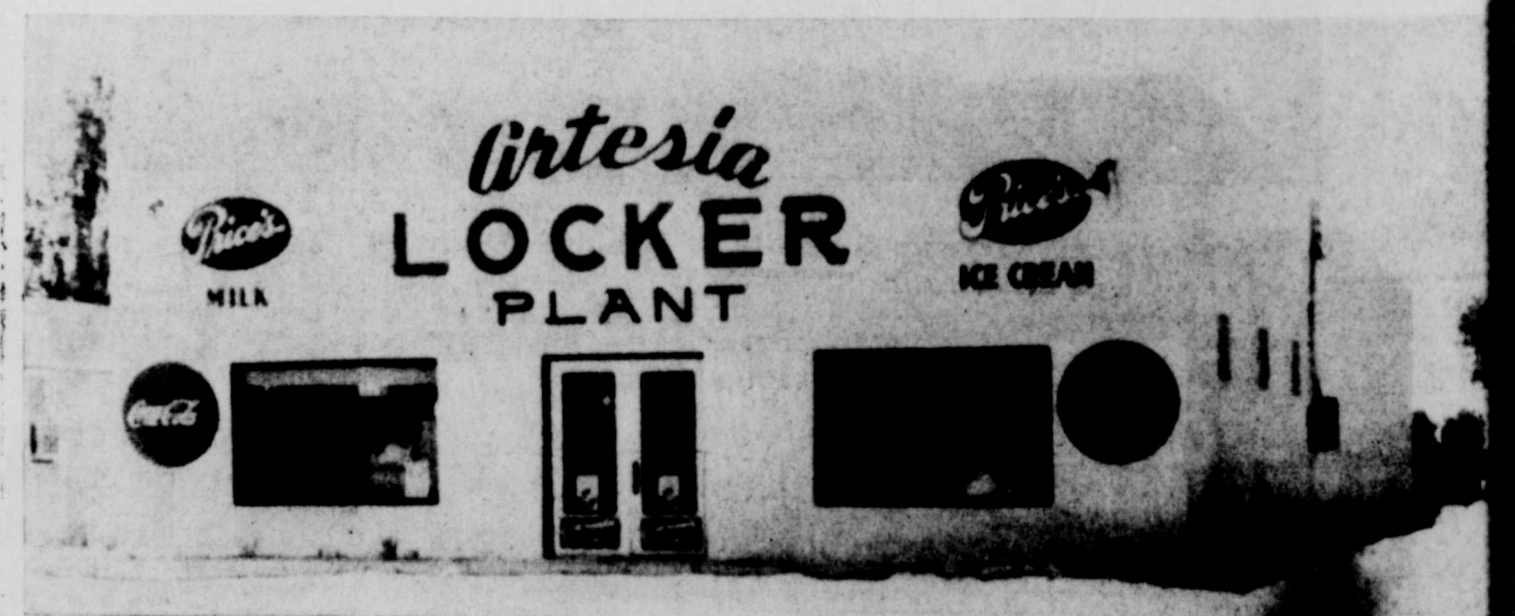
THIS is the exterior of the Artesia Locker Plant, 302 South 13th.
