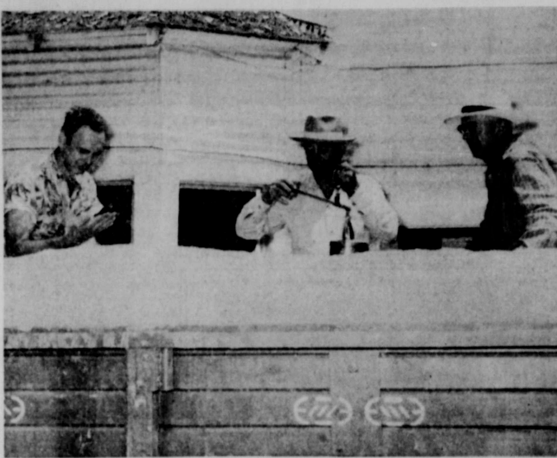
ELEVATOR'S FIRST LOAD—Gene Brothers, left, and H. B. Urban, right, watch D. W. Hart of the Equity test the first load of wheat brought to the Perryton Equity elevator this season. The wheat was Early Triumph, grown by Bob Urban on irrigated land 19 miles south and three miles west of Perryton. The wheat tested 61.5 and had 11.40 moisture. Urban estimated it was making better than 30 bushels per acre. The Urbans plan to harvest about 140 acres of irrigated wheat and about 500 acres of dryland wheat this year.
