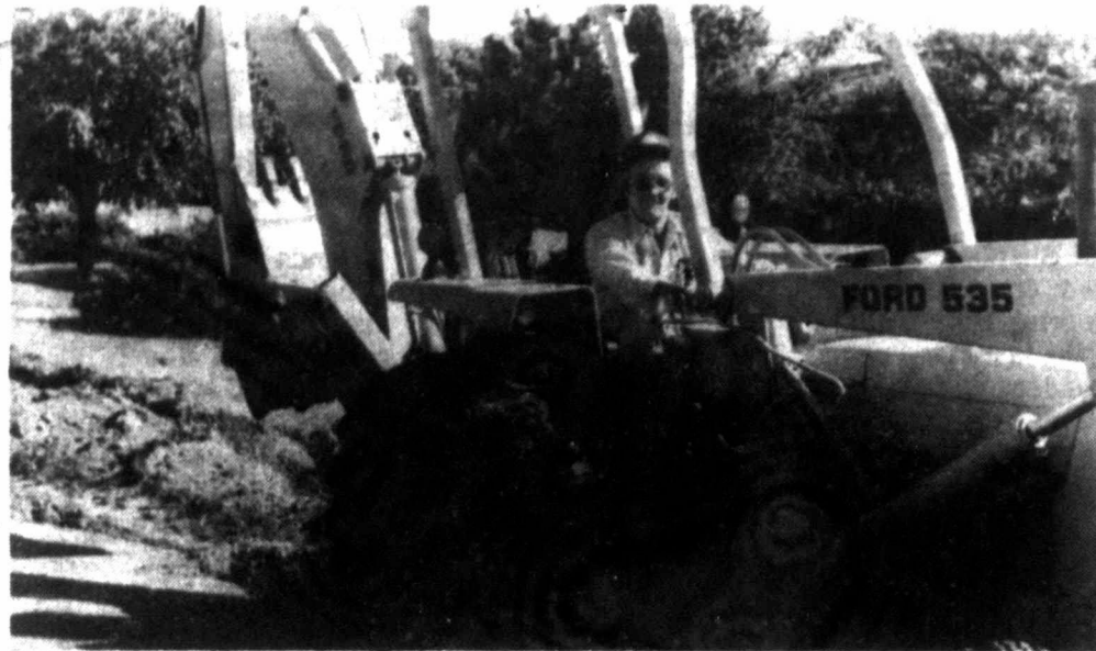
GOOD NEWS for residents served by water lines running up Elm and 13th Street where there has been little or no pressure for some time. Water Superintendent Buzz Rich has begun laying 1,200 feet of new six inch water main. "This has been a pet project of Buzz's and we finally managed a few extra dollars to do it with," City Manager Ray Mason commented. He also noted there will be a new fire plug installed at the corner of 13th and Elm Street.
