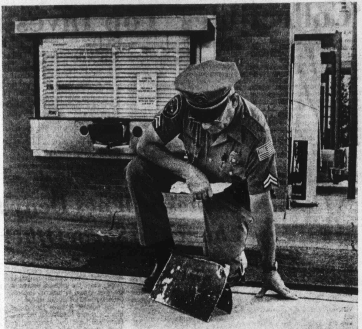
BANK BOOTH BOMBING — Lubbock Police Cpl. Emmett Caddell investigates the remains of a money deposit tray ripped from a teller booth when a "pipe bomb" exploded late Wednesday or early this morning at Security National Bank,
