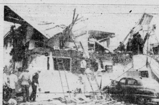
BLAST WRECKS APARTMENT BUILDING—This was the wreckage of a North Hollywood, Calif., apartment building after a shattering explosion, believed caused by escaping gas, blew out second-story walls and half of roof.
